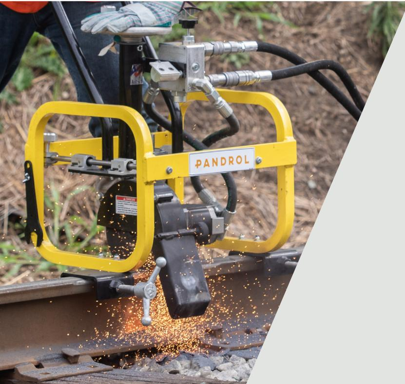
The Pandrol Head Wash Grinder is used to prepare the rail for head wash repair aluminothermic welding.
